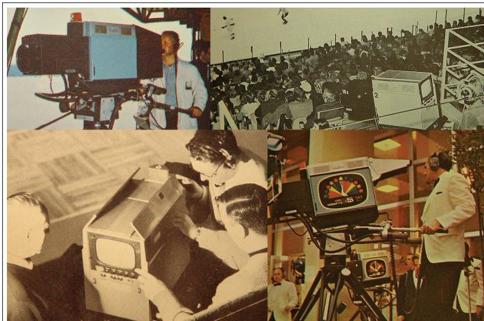
Figure 4.16 Within a couple of years, RCA responded to the PC-70 with its TK-44. These camera heads were approximately 50 lbs., and they made remotes much easier to accomplish. While both ABC and CBS made extensive use of the PC-70, there were a number of trucks that used TK-44s.
